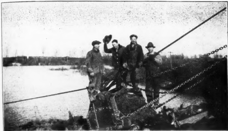
A Bucket Load and Plant Employees at Morristown
